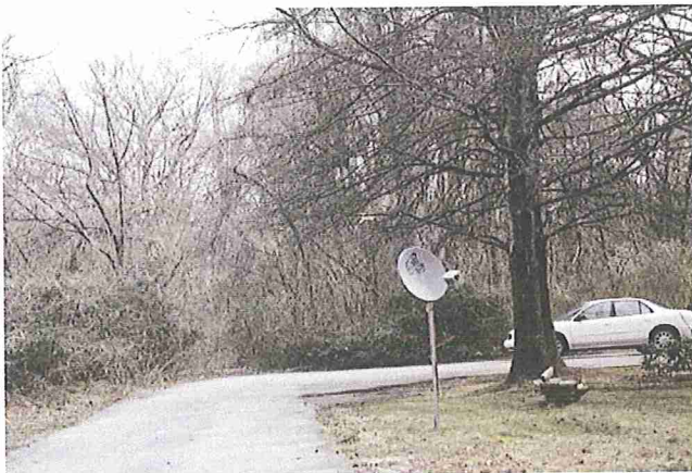
SITE – Stone Pointe Apartments Shadow Wood Drive Clinton, SC Facing east at end of Shadow Wood Drive Duplex is on right
