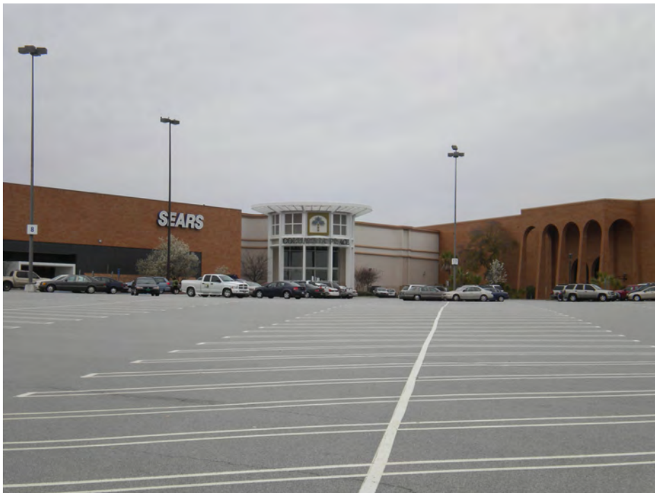
Nearby Columbia Place Mall is anchored by Sears, Macy's and Burlington Coat Factory.
